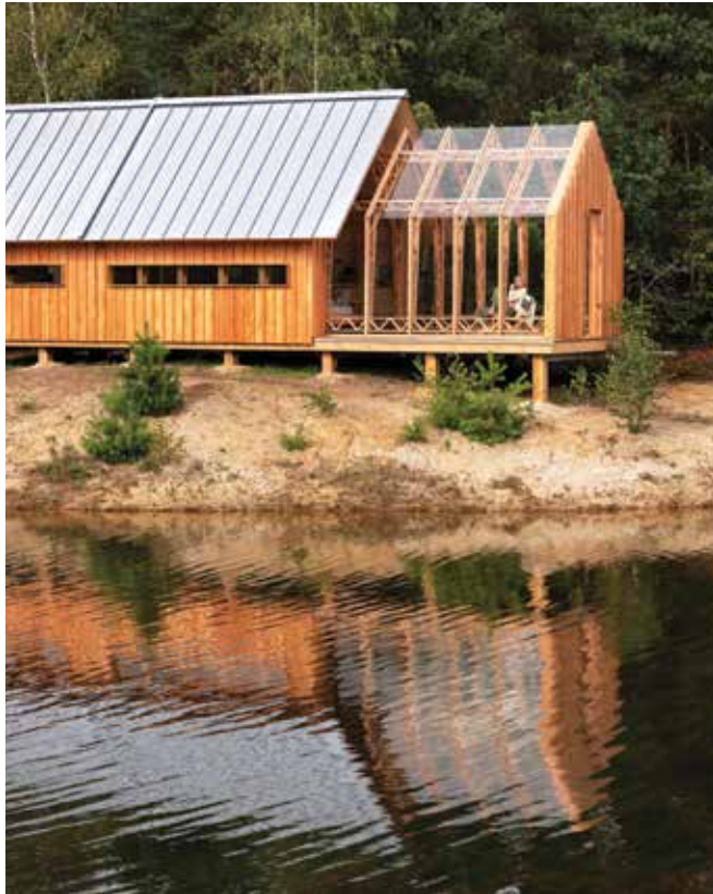
Above: The cabin's shells slide open, allowing people to transform the cabin according to their own needs. 小屋的外牆非常容易推開，屋主可自行安排兩層牆壁的位置，以適應各種需求。
